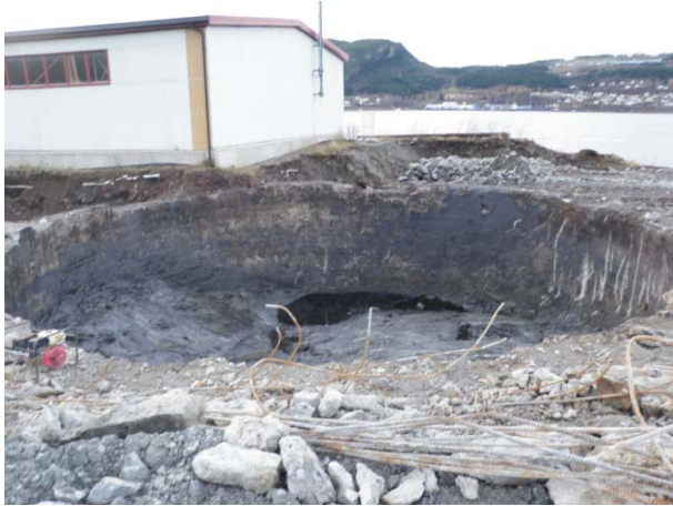
Kreosottank ferdig rensket.
